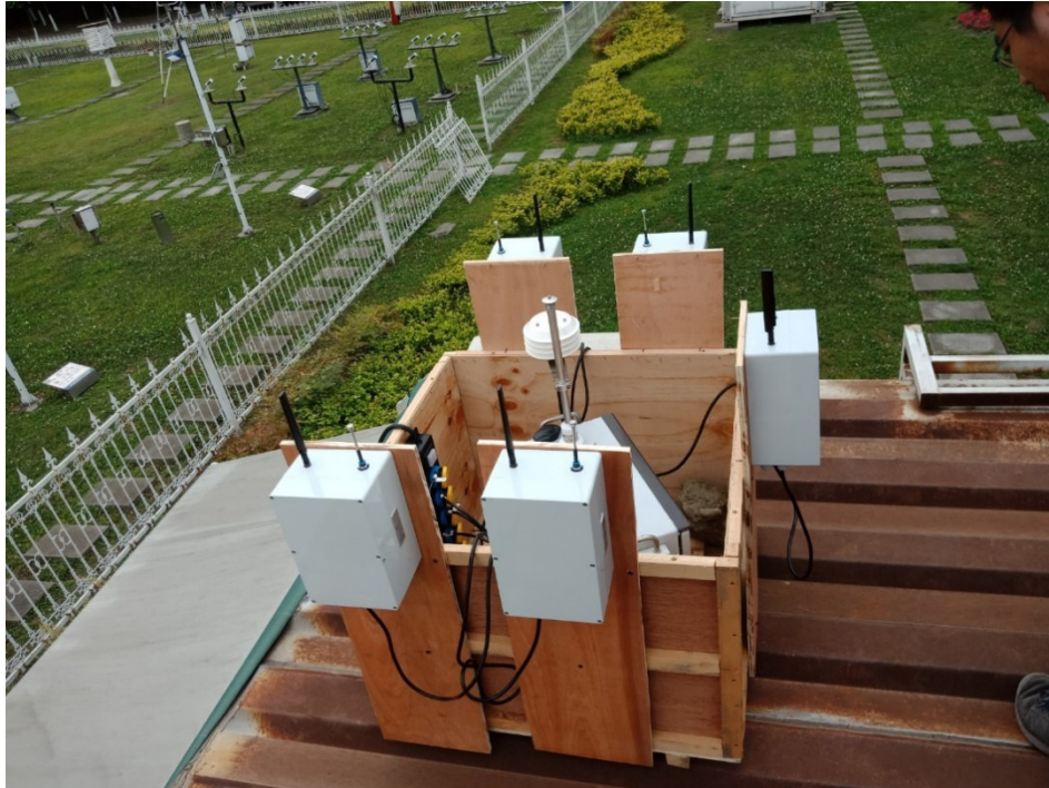
Figure 5: Similar to the intercomparison setup at Augsburg measurement site the installation at Chengdu was carried out (Picture: GRIMM)
